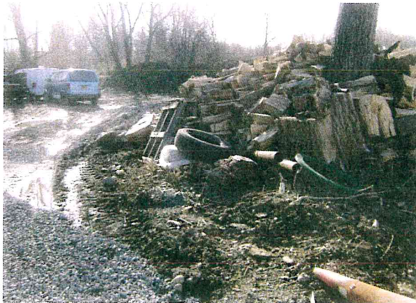
13. New berm and site grading
