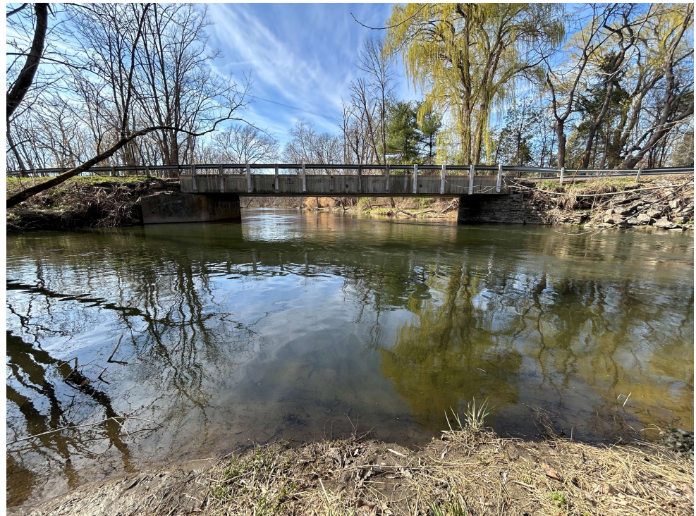
Existing Upstream Elevation (looking Northwest)
