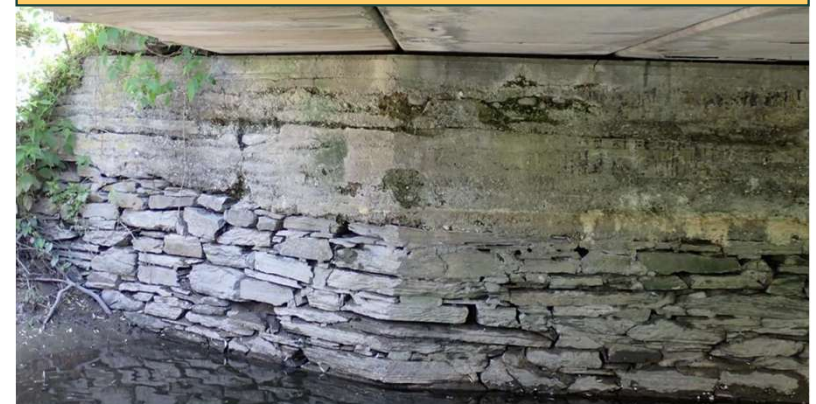
Missing Mortar and Stones
