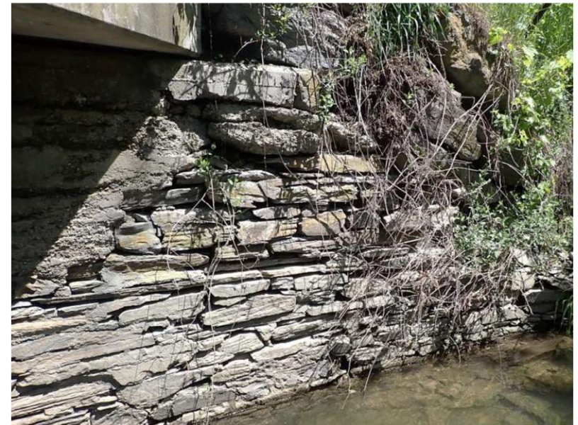
Missing Mortar and Stones
